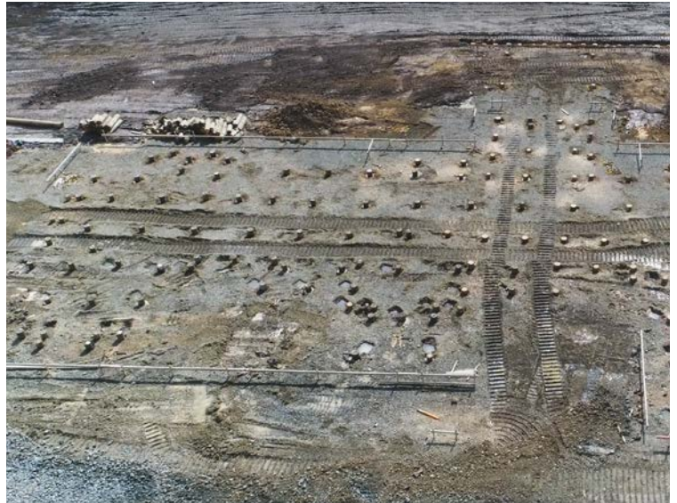
Photos courtesy of Markovina Pile Driving
