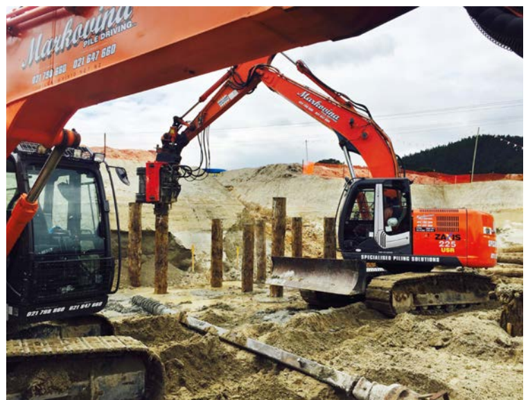
Photos courtesy of Markovina Pile Driving
