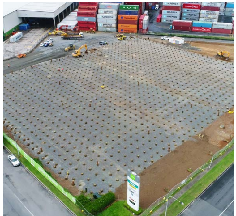
Photos courtesy of Markovina Pile Driving
