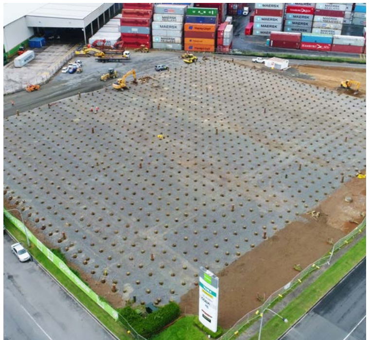
Photos courtesy of Markovina Pile Driving
