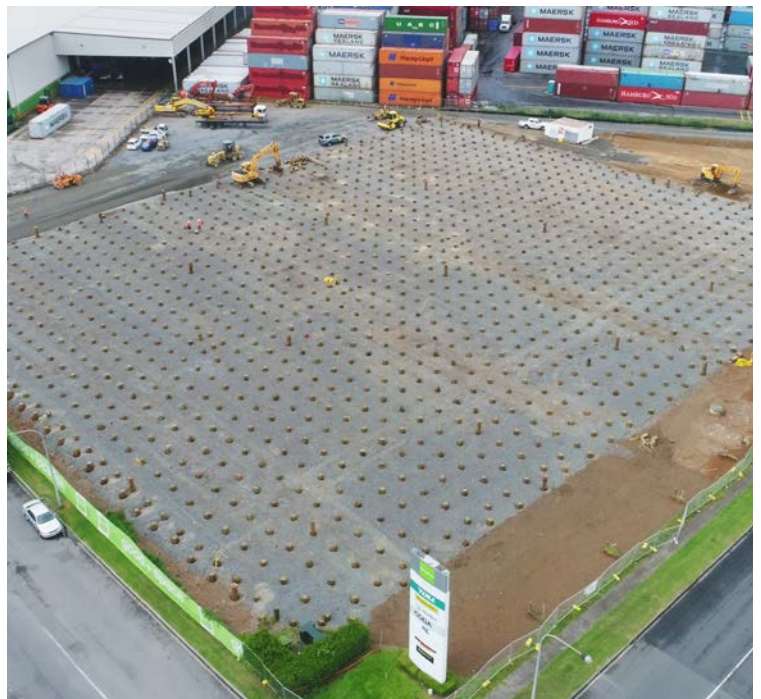
Photos courtesy of Markovina Pile Driving
