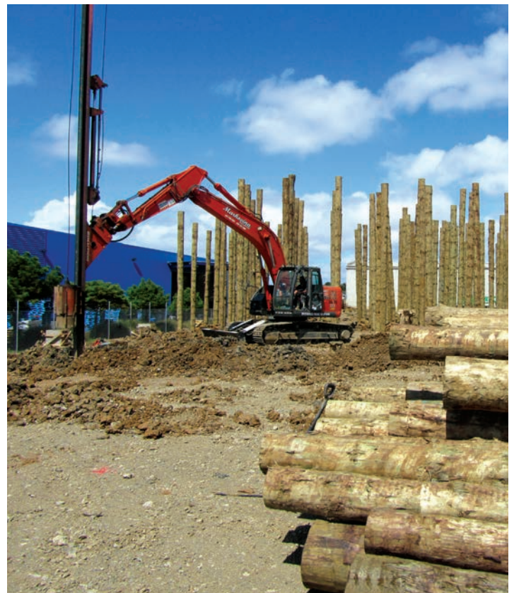
Installation by Markovina Pile Driving
